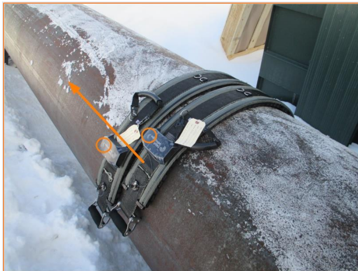
Figure 3: 16" and 18" Piezo-Tools ready for installation on a 36" Schedule 40 pipe
