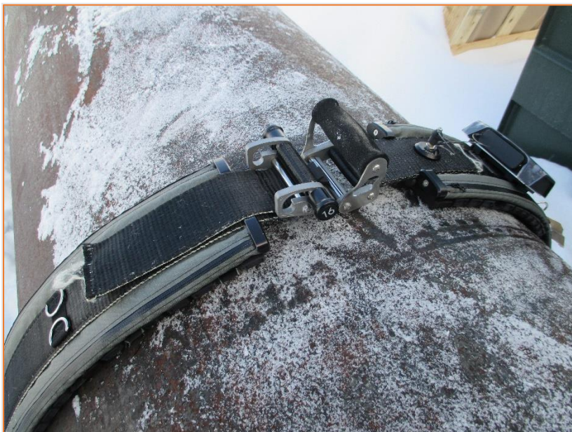
Figure 5: Initial collar engagement at TDC of the pipe
